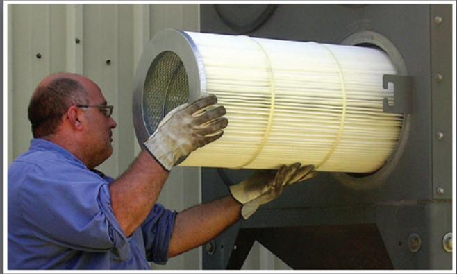
require the additional use of a costly HEPA filter to ensure a safe breathing environment. This adds to overall filter cost and system upkeep.
